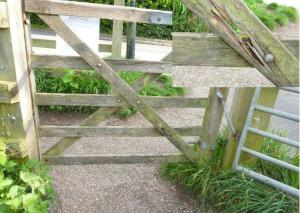
**Footpath 4:** This foot path remains the most challenging to maintain due to the overgrowth of weeds and nettles along the length of the path from the end of Common Lane through the pony field. This path is little used which makes keeping it clear problematic. The style at the Common Lane end (Photo 3) is becoming unsafe because one of the upright legs is rotting (Photo 3 insert) and should be repaired.
