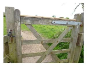
**Footpath 2:** This path runs across Chapmans field along the river to Hemingford Grey footpath 12. The gate at the Quiet Waters end has been repaired recently by the addition of a capping bar to the top of the gate (Photo 1). The other two gates along this path have been replaced and are in good order.
