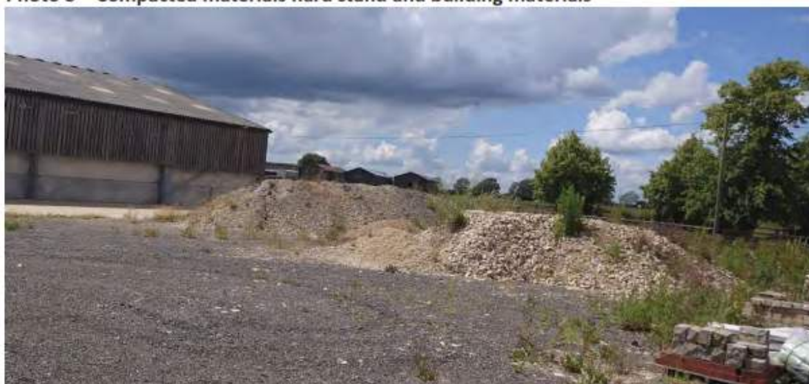
Photo 8 – Compacted materials hard stand and building materials
